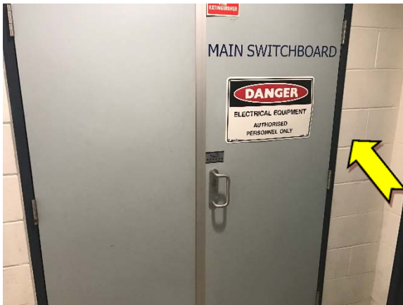
Photo 3. Interior, throughout (except courts), walls – suspected lead-containing white upper paint system.
